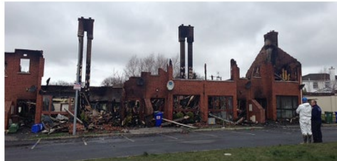
Figure 2. Fire stopping / compartmentation omitted.
