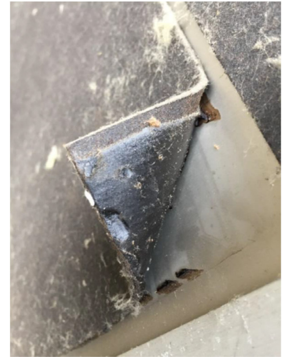
Bitumen sheeting on the back of the sheet metal panelling
