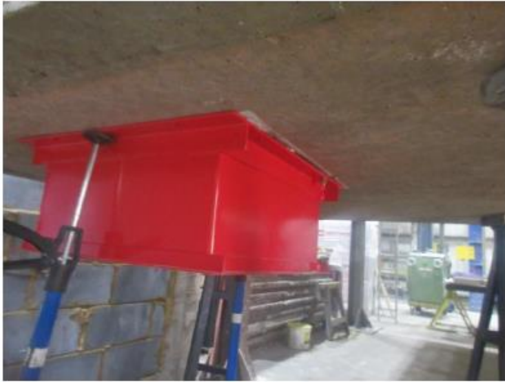
Photo 3. Installation of chute to underside of concrete slab.
